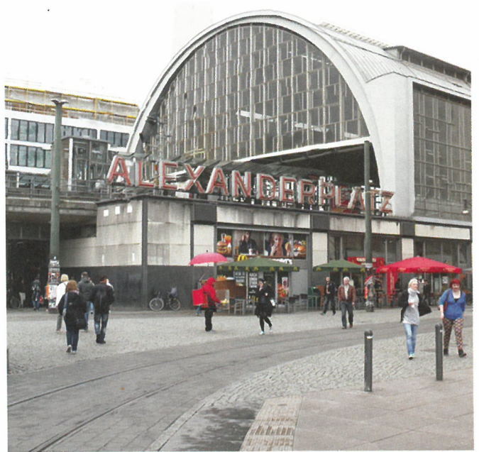
Figure 6.23: Image with cables removed.
